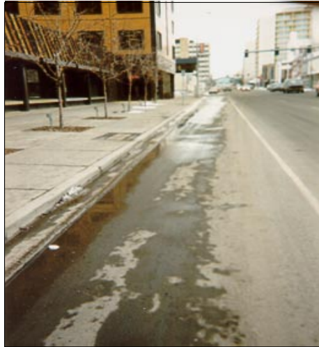
March 25, 1999. Streets and sidewalks are bare, some ponding along curbs (5th Ave.)
