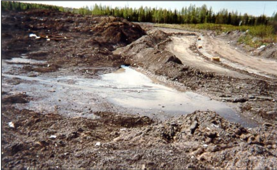
Entrance Pond, Dry V-Ditch - TU01
