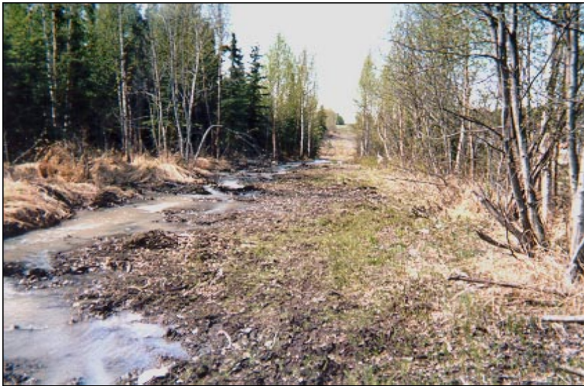
Overflow from Infiltration Area
