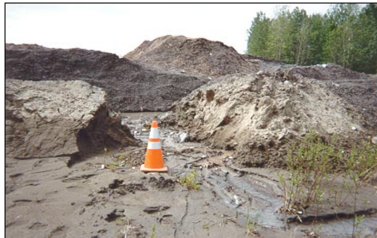
Berm Failure above Pond (TU02) - (6/8/99)
