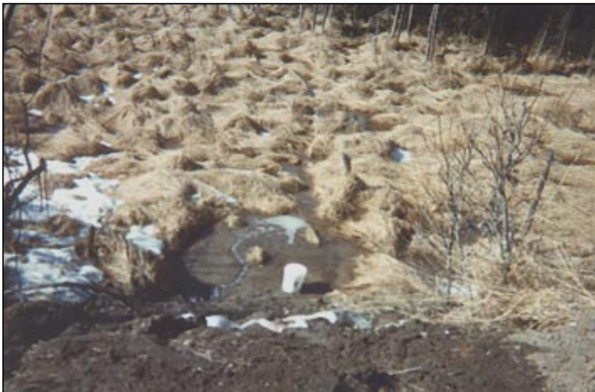
Access Ramp Flow into Swamp (TU06)
