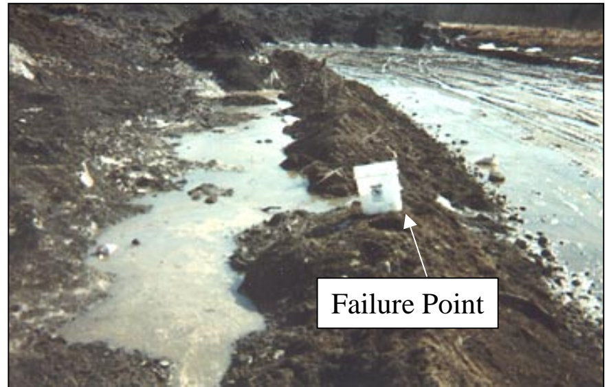
Top of Access Ramp
