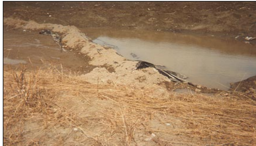
Top of Access Ramp Berm
