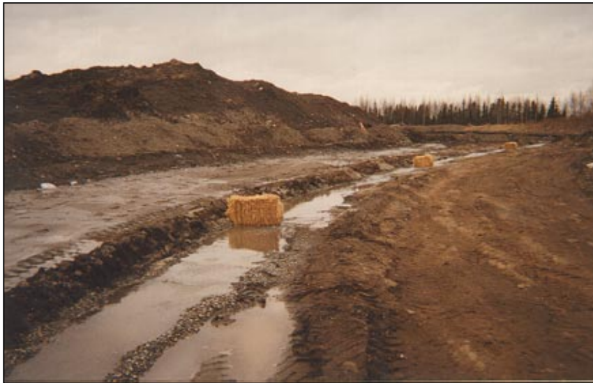
V-Ditch Up Access Ramp
