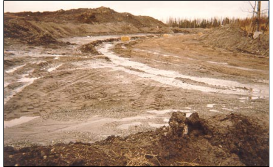
V-ditch Up Formed Up Access Ramp
