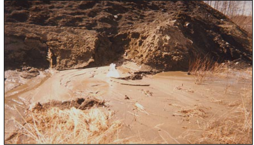
Berm Above Pond (TU02) - (4/28/99)
