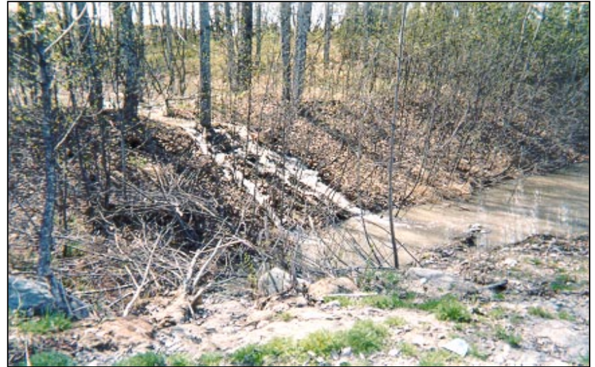
Infiltration Area Overflow into Tudor Ditch
